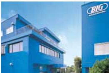
● Head Office FA Factory
